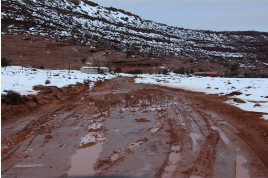
Image provided by San Juan County
